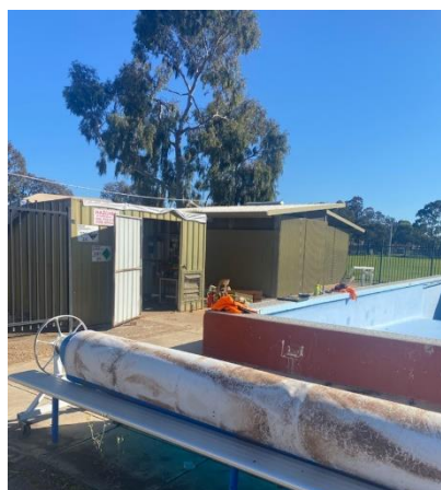
Shed being emptied, ready for replacement
