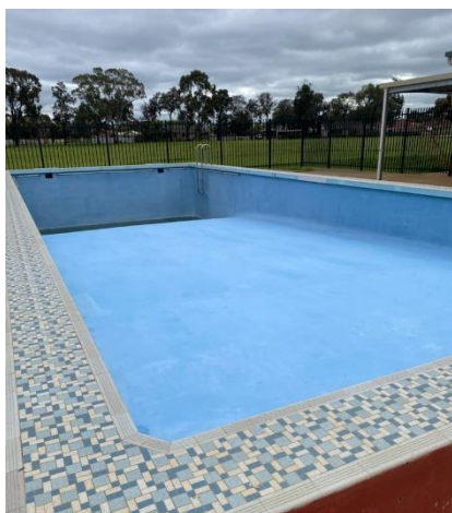
Pool emptied for repairs
